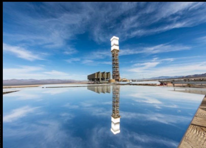
BRIGHTSOURCE ENERGY INC
